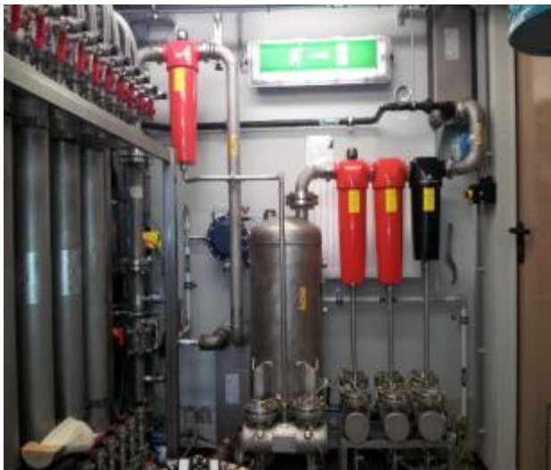
Figure 8: PFD Carborex® MS system and picture of membrane container
